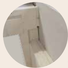
Multi-layer refractory insulation with light-weight refractory bricks
